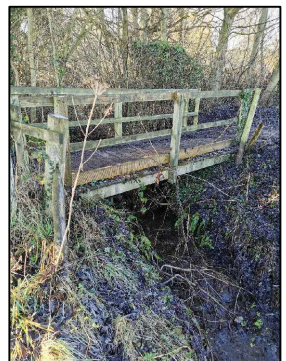
PHOTO 2 - EXISTING TIMBER FOOTBRIDGE
